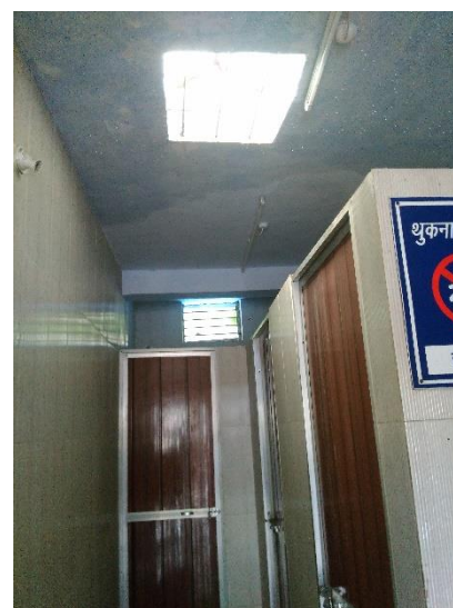
Photo 4: Neat and Clean, Well Light Public Toilet Complex
